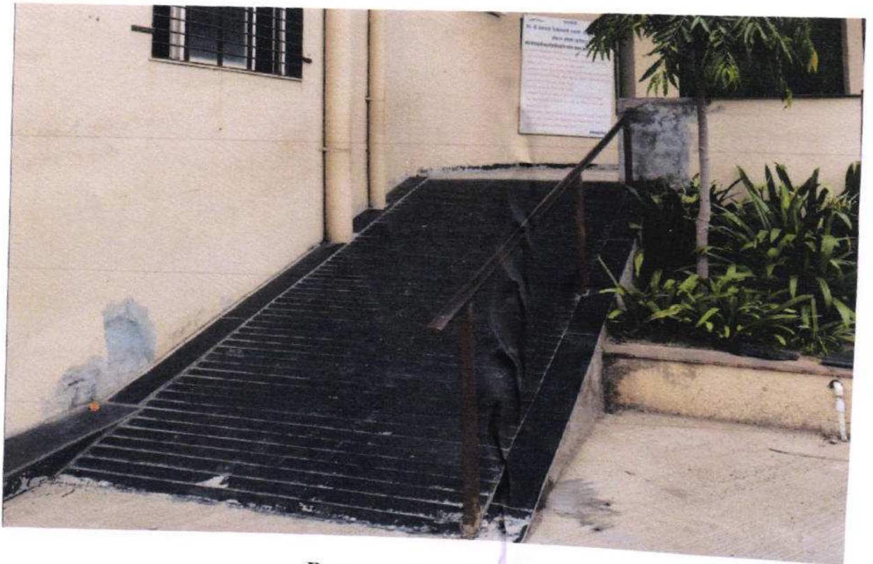
Ramp at science building
