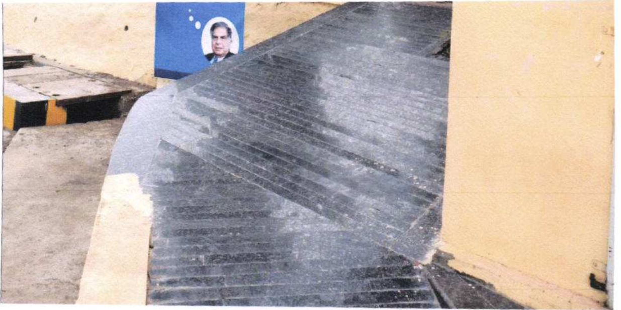
Ramp at main building
